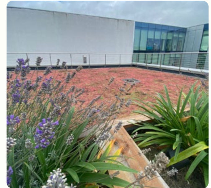
Figure 2-13: Green Roof on the Observatory in 2025.
