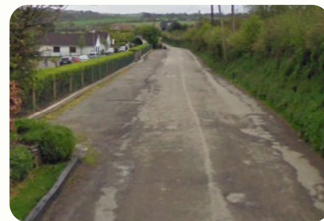
Figure 5-4: Before construction, the area consisted of impermeable surfaces in tarmac. Source: Google Maps, 2024
