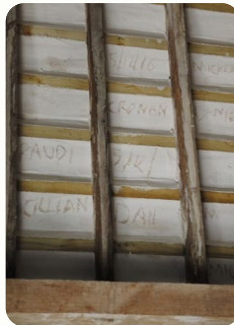
Figure 6-11: No breathable felt used. Source: Anna Meenan, n.d..
