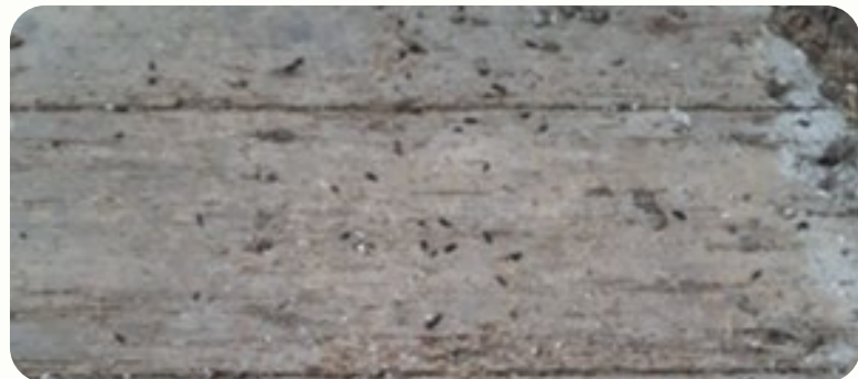
Figure 6-6: The interior of the building with bat droppings accumulated on the first floor. Source: Anna Meenan, 2021
