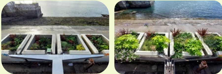
Figure 5-12: Rain Garden when first established with channel cover in place (left) and after establishment with channel cover removed (right). Source: Cork County Council, 2023
