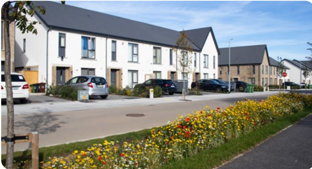
Figure 3-9: Example of planting at Parkleigh - Seven Mills (Tile 1). Source: Cairn Homes, 2025
