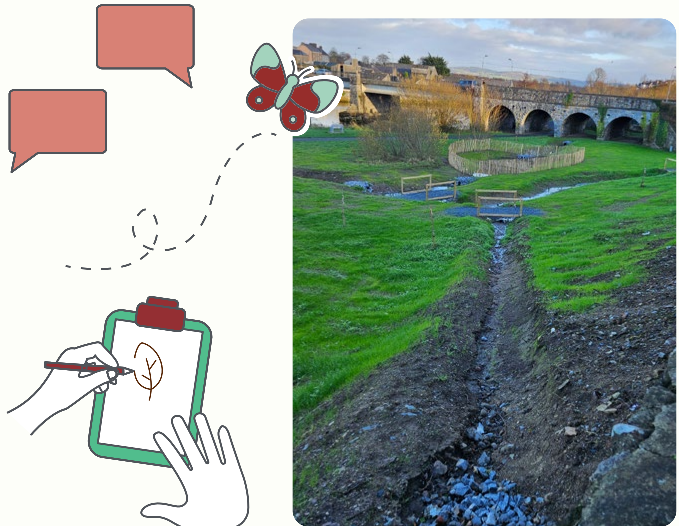
Figure 7-8: Road runoff is discharged directly into a grassed conveyance strip that flows into a newly planted swale below. Source: Ben O'Keeffe, 2024
