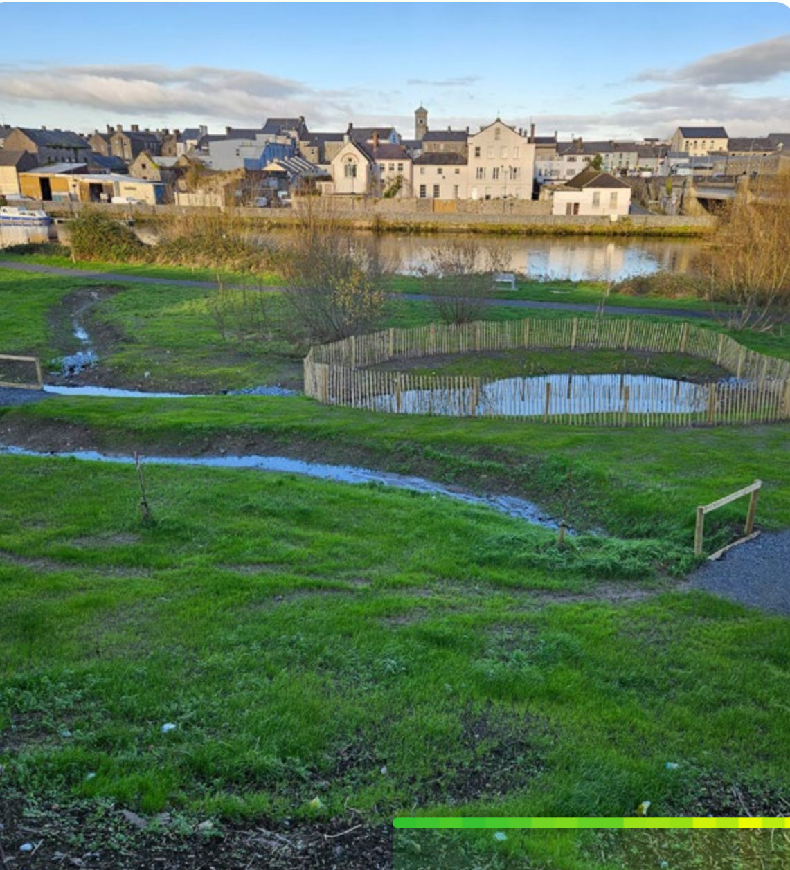
Figure 7-1: Swales and infiltration pond as nature-based solutions to improve water quality of road runoff. Source: Ben O'Keeffe, 2024
