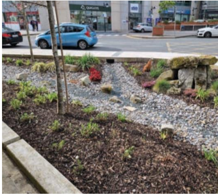
Fig. 12: Rain Gardens in Pollerton Road, Carlow (Igoe et al., 2025)
