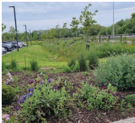
Fig.11: Dry Swale - Min Ryan Park, Wexford (Igoe et al. , 2025)
