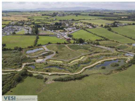
Fig.4: Aerial view of Dunhill's Integrated Constructed Wetland (ICW) (VESI Environmental, no date)
