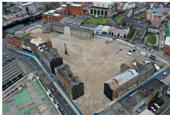
Figure 2 Opera Square project end of Contract A (Demolition and Enabling Phase)
